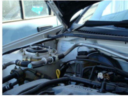
Early 2000s: Stiff firewall and sides of engine bay supporting edge of bonnet. Minimal clearance between suspension tower/engine cover and bonnet.
